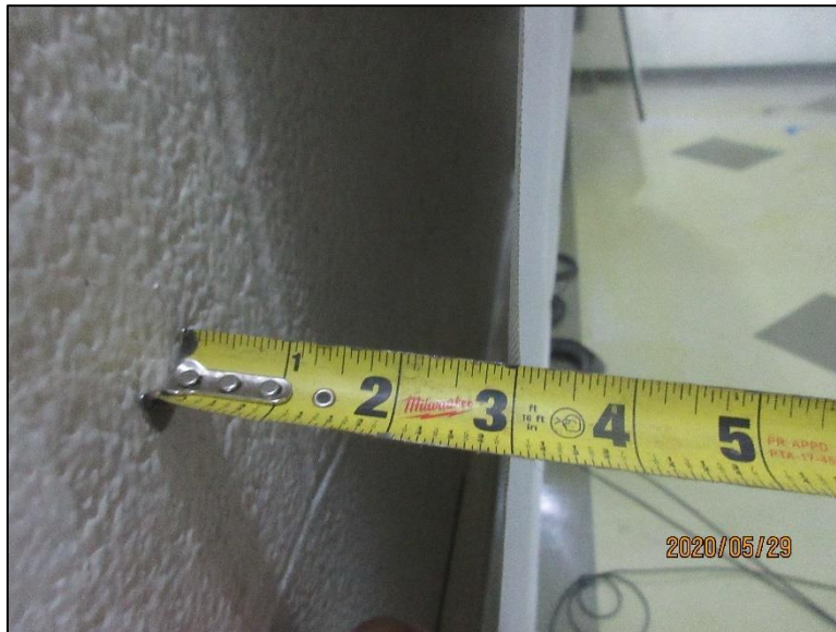
Photo No. 2 Side View of Installed Test Specimen
